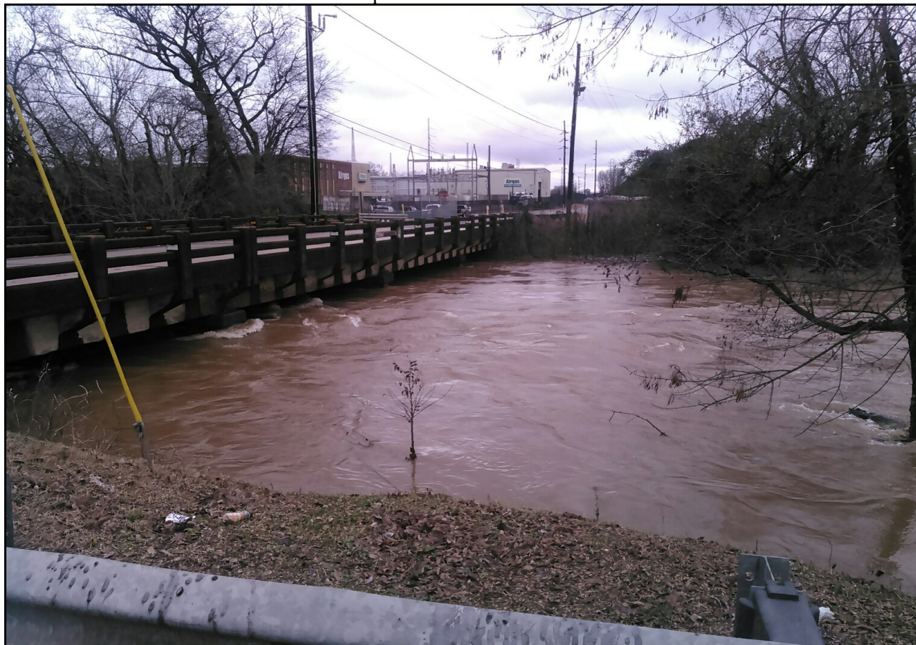
Figure 2. Valley Creek Water Flow Under 18th Avenue Bridge
